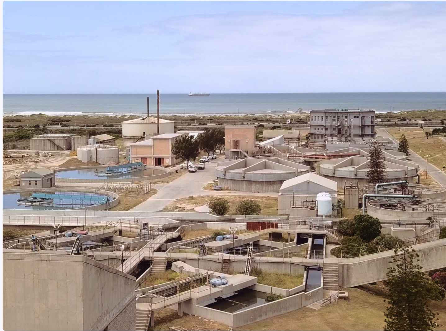
Above and previous page: Aerial view of the Fishwater Flats Waste Water Treatment Works in Nelson Mandela Bay Metropolitan Municipality. Credit: Charles Meadows for REEEP
