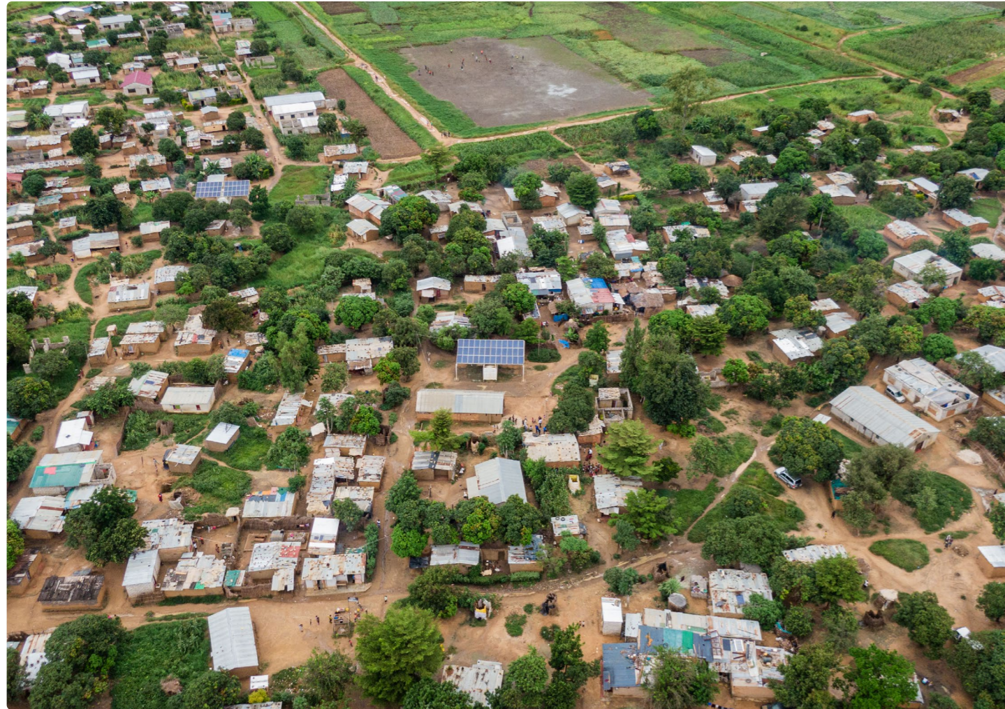
A Standard Microgrid mini-grid installed in the centre of Ngewere, on the outskirts of Lusaka, Zambia. Credit: Jason J Mulikita
