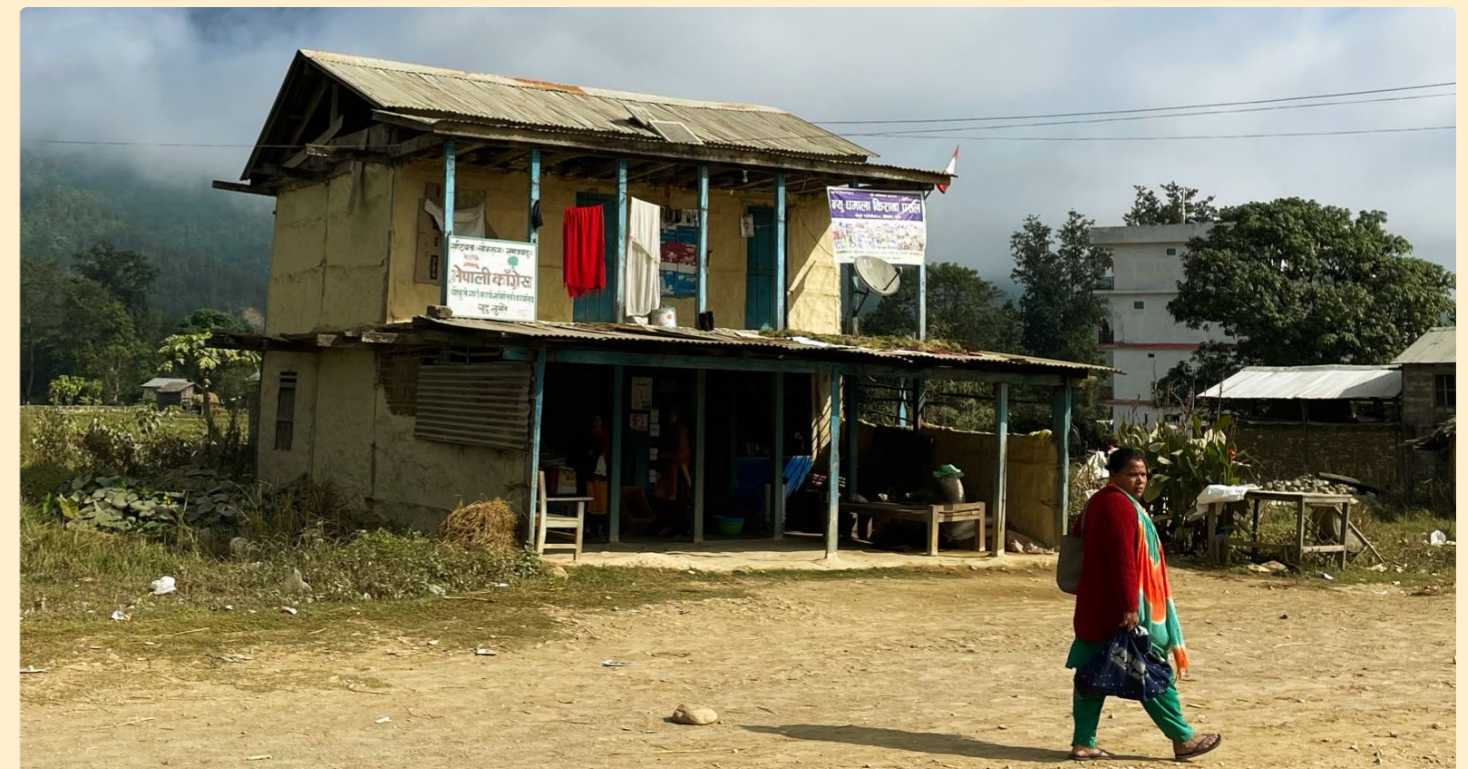
Left and above: A solar farm powers the remote village of Gutu, in the province of Karnali, Nepal. Credit: Stewart
