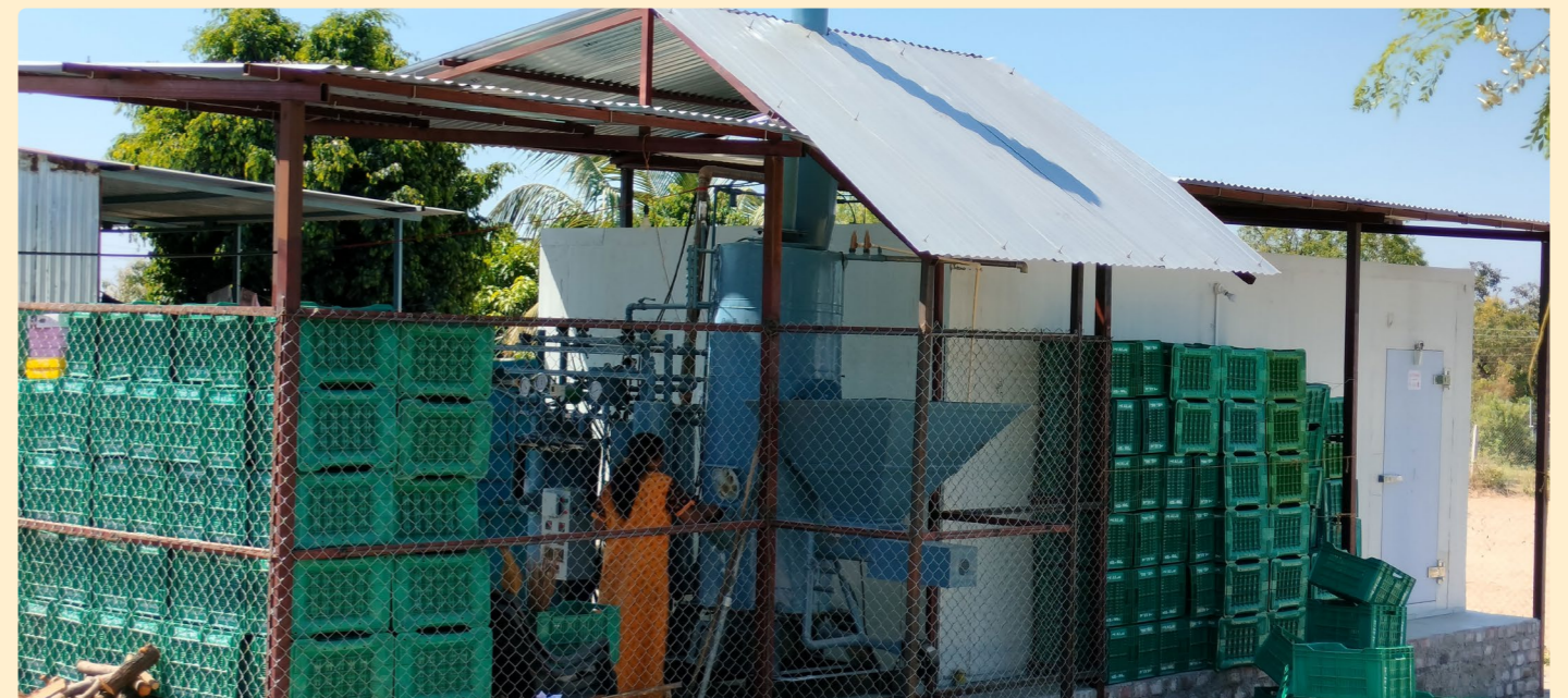
Left: A worker harvests avocados which will be kept fresh longer through SokoFresh's cold storage hub near Nairobi, Kenya. Credit: Redbunny Above: Cold storage solutions at PFAN-supported project New Leaf Dynamic Technologies in India. Credit: New Leaf
